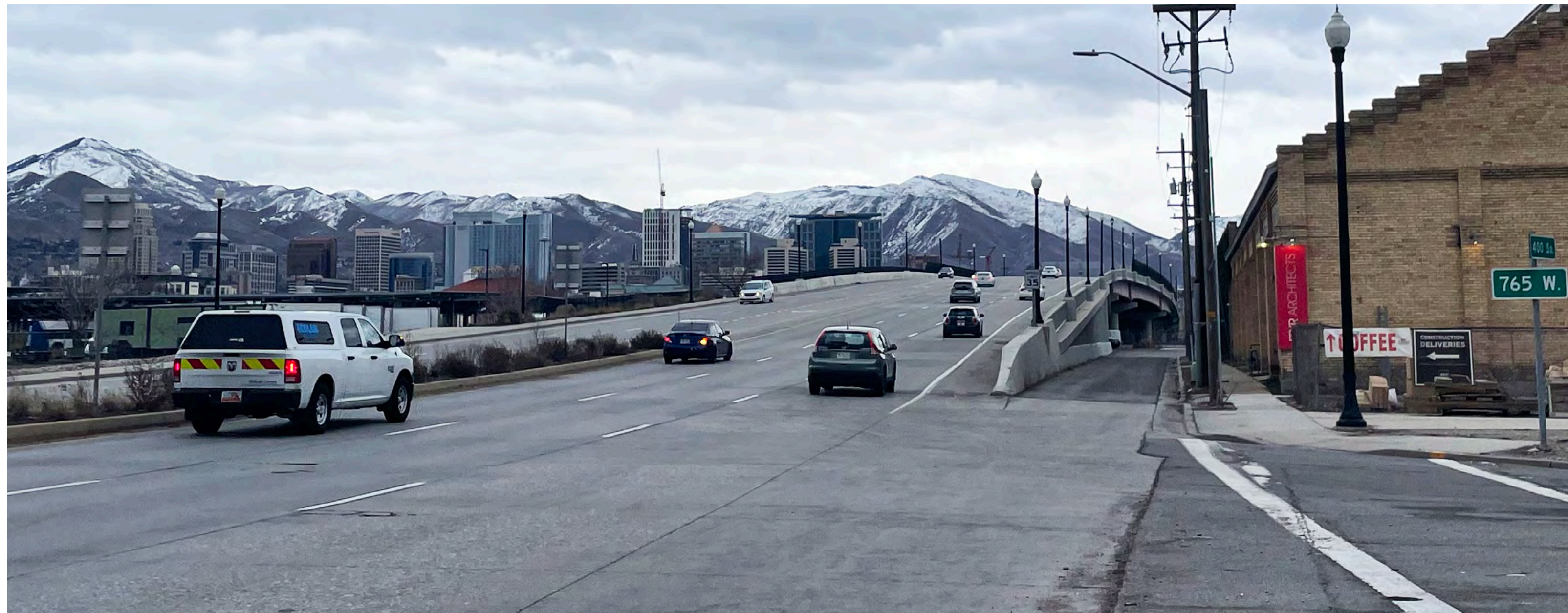
Approaching Viaduct from west; the crosswalk seen in the lower right corner of this image will connect to a new multi-use trail on the south side of the bridge.
