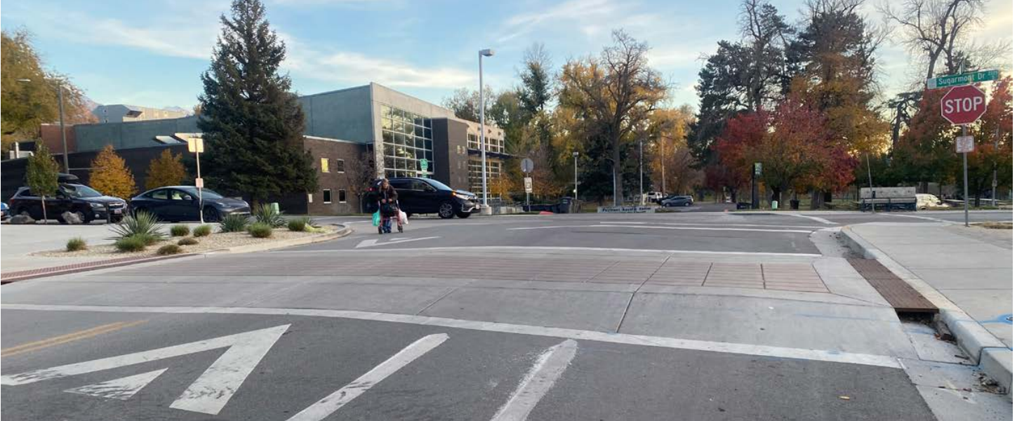
Raised crosswalk along the S-Line Trail in Sugar House, Salt Lake City, UT
