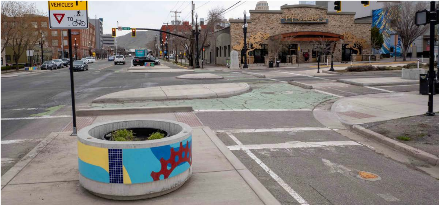
Full Protected Intersection (300 S 200 W) in Salt Lake City, UT
