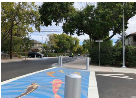
Asphalt raised intersection in Palo Alto, CA
