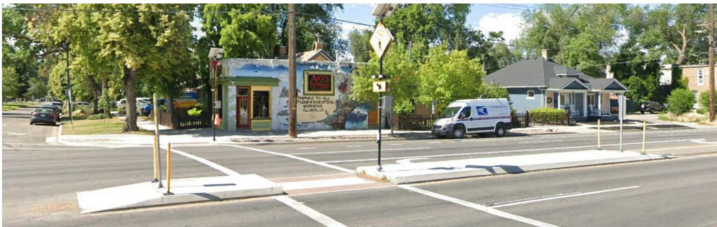
Median refuge with RRFB at 800 S 600 E in Salt Lake City, UT. Source: Google Earth
