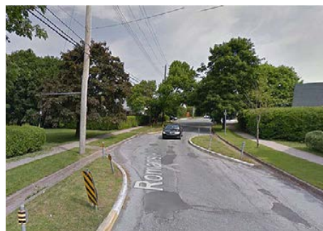
Chicane designed to retain drainage Source: FHWA via Google Street View
