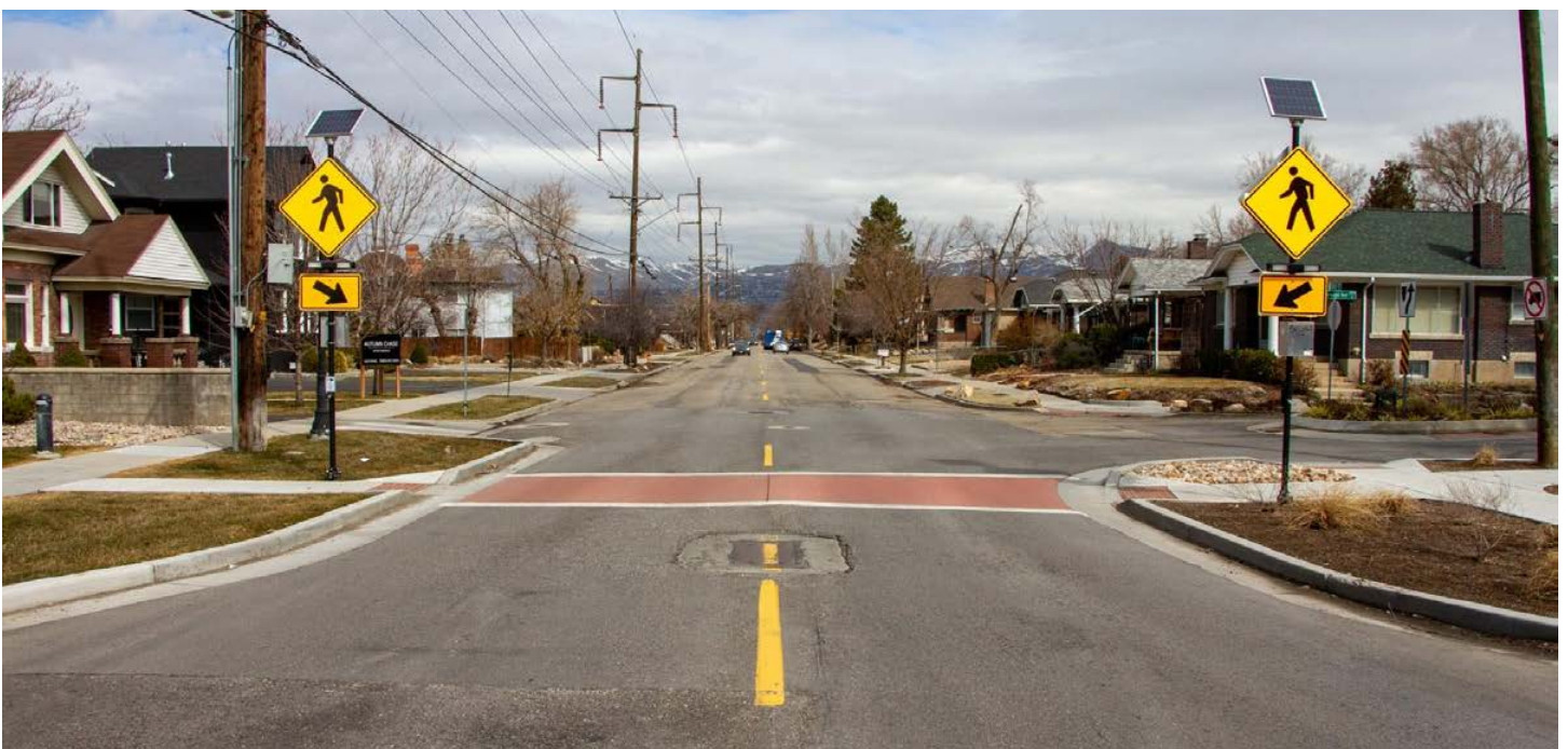
Choker with crosswalk (horizontal deflection) at Ramona & 900 E in Salt Lake City, UT
