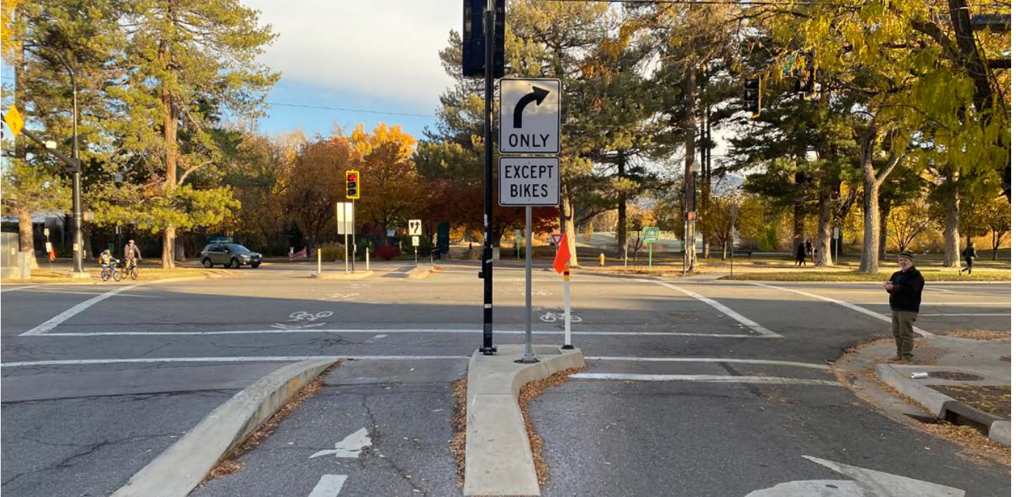
Toucan crossing at 1300 S & 600 E in Salt Lake City, UT. Source: Google Earth
