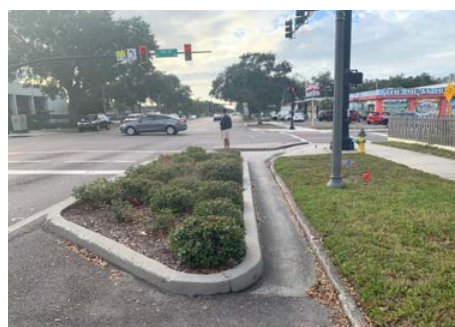
Floating curb extension in St. Petersburg, FL
