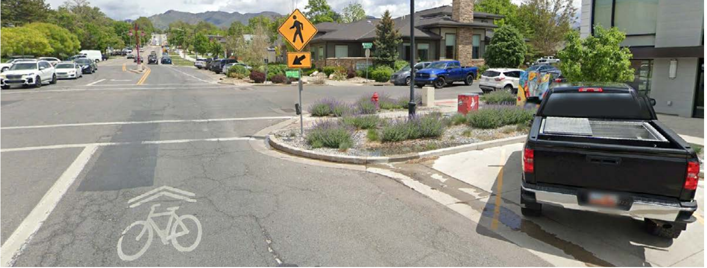
Curb extensions at 900 S & Lincoln St in Salt Lake City, UT. Source: Google Earth
