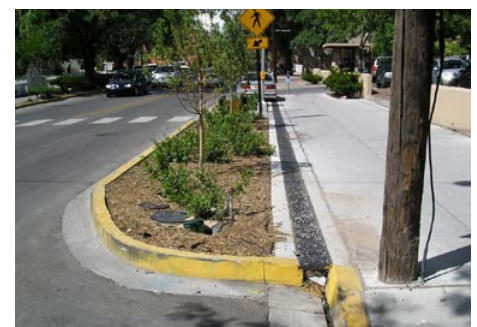
Curb extension with chase cover Source: NACTO
