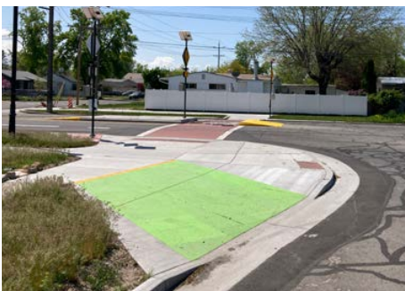
Bike ramp in Salt Lake City, UT (1000 N 1300 W)
