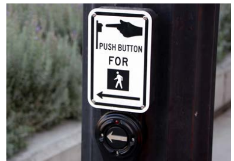
RRFB push button signage
