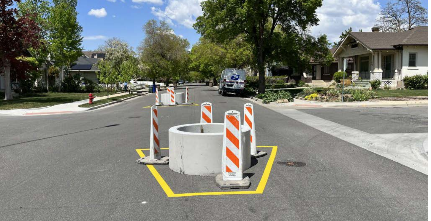
Traffic calming ring pilot project at 1000 E & Ramona Ave in Salt Lake City
