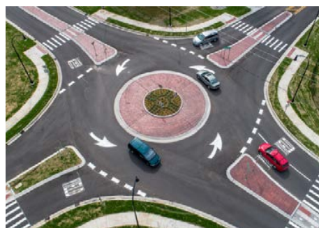
Roundabout with brick detailing
