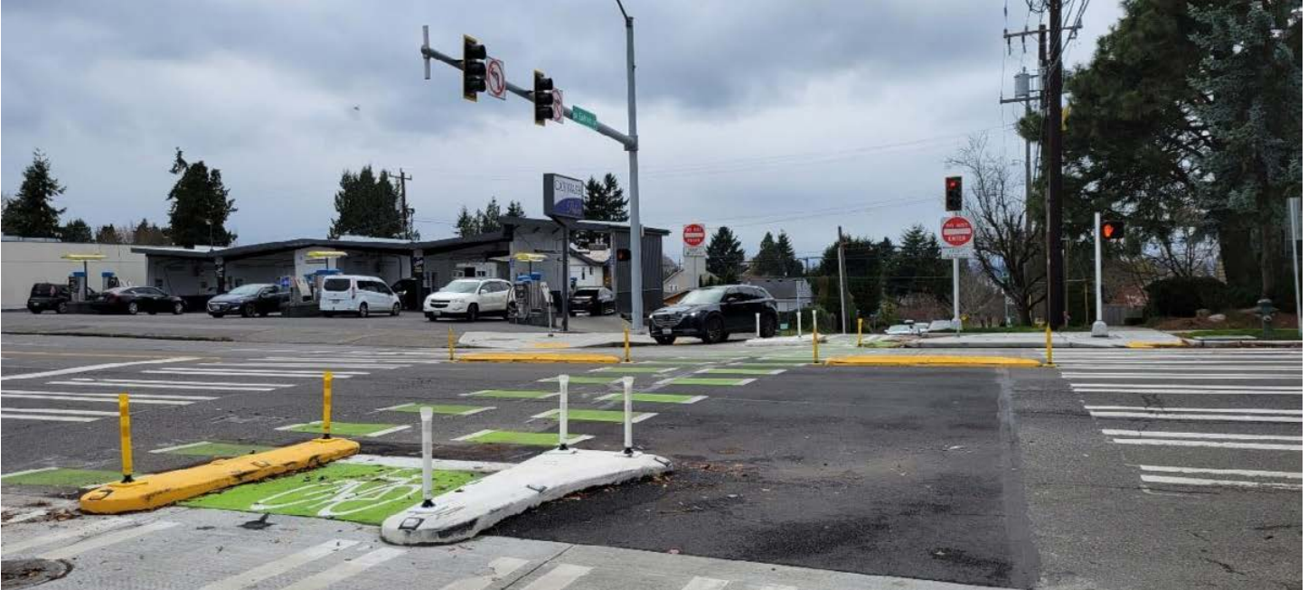
Intersection crossing markings and protected waiting area in Seattle, WA
