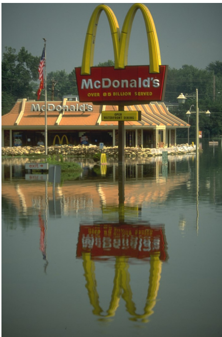
Photo Courtesy of Andrea Booher/FEMA Photo
